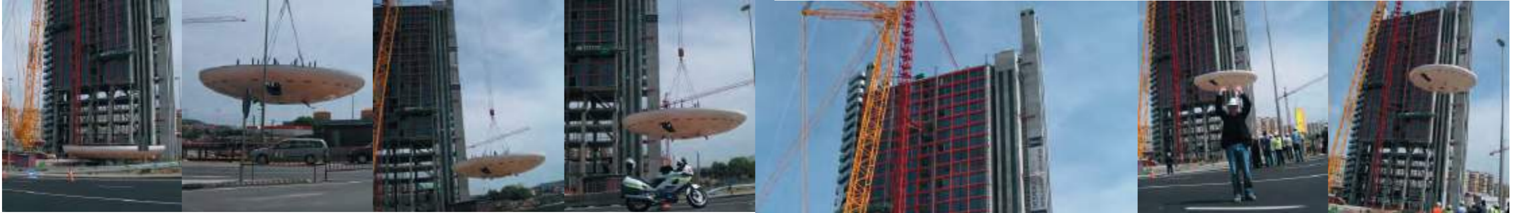
The hoisting of the lower part lasts 3 long hours, 30 tonnes at a height of 105 metres.
