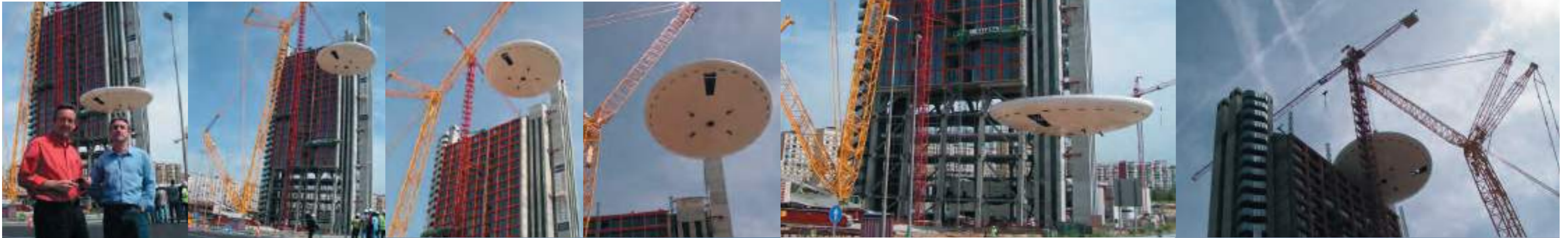
The hoisting of the lower part lasts 3 long hours, 30 tonnes at a height of 105 metres.
